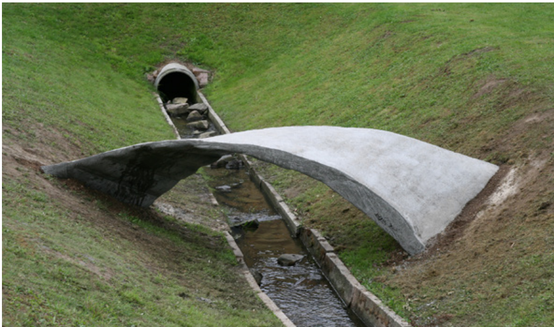
Abb. 19 Brücke Concretum (Carmen Rist-Stadelmann, 2010)
